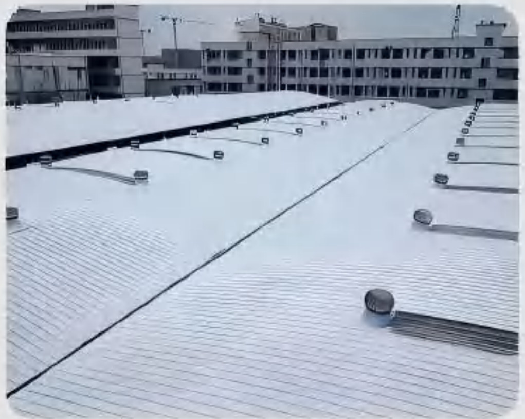
Anti-Corrosion Project: 20,000 sqm
